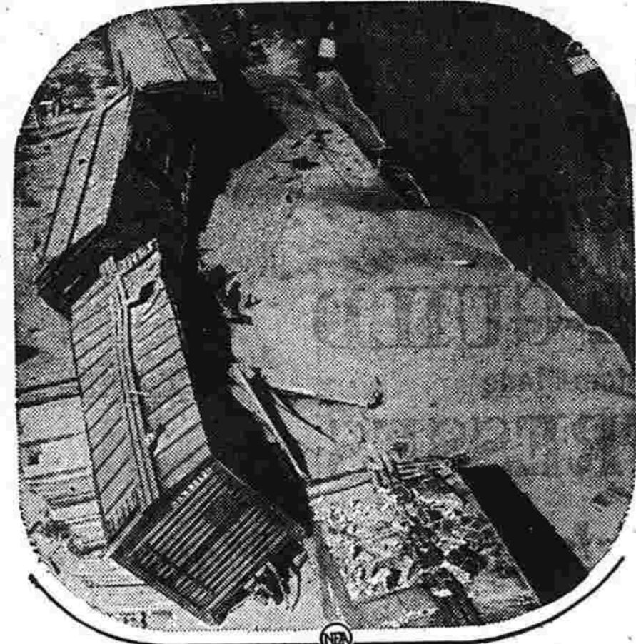
This picture shows what happened when an elevator containing one million bushels of wheat exploded at Des Moines, Ia. A half-million bushels spilled out of the elevator when a dust explosion blew out the side walls of eight of the 10 bins. Two freight cars were literally lifted up and hurled aside.
